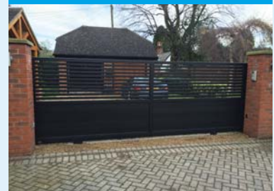
GARITA - SLIDING GATE
